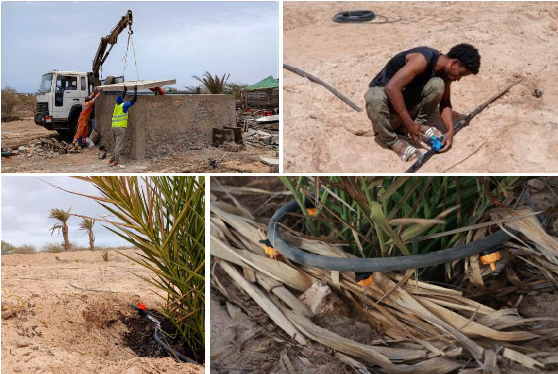
Figure 10 – Rehabilitation of the water deposit (top left) and installation of the drip watering system in the oases of Beirona (top right). The new system increased the water efficiency and reduced time and costs (bottom).
